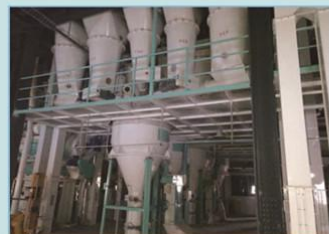
Feed Line in Installation
