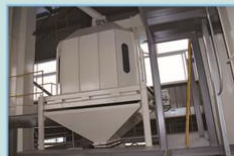
Installed Cooler 安装完毕
