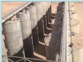
Silos in Feed Line
